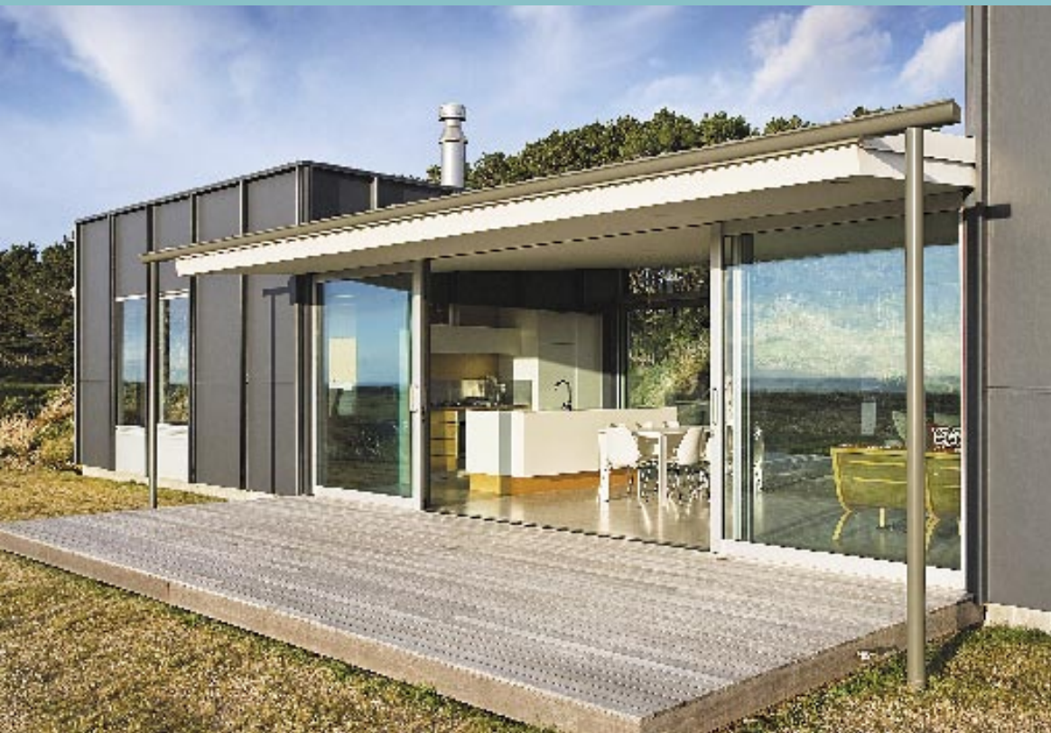
ABOVE: Looking along the western elevation, with the deliberately “oddball” extended guttering on the roof over the terrace.
