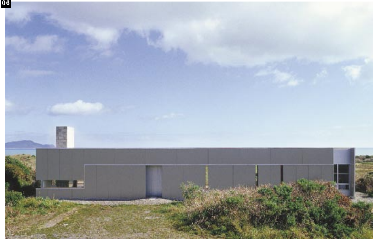
06 South elevation of Paetawa House.
